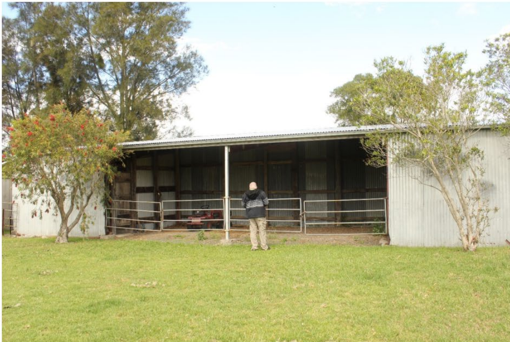
Figure 18: Showing detail of recent barn construction. The barn appears to have been constructed using recycled materials from an earlier barn of structure (as was indicated by Melinda on site).
