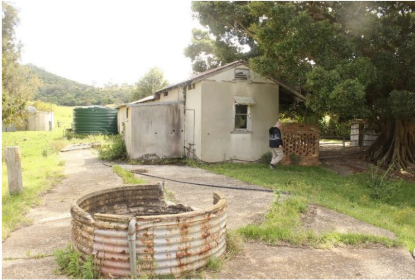
Figure 13: Southern façade of dairy building. Note the western addition, slab areas surrounding, and corrugated circular water trough. Note also the substantial and established Fig to right of building.
