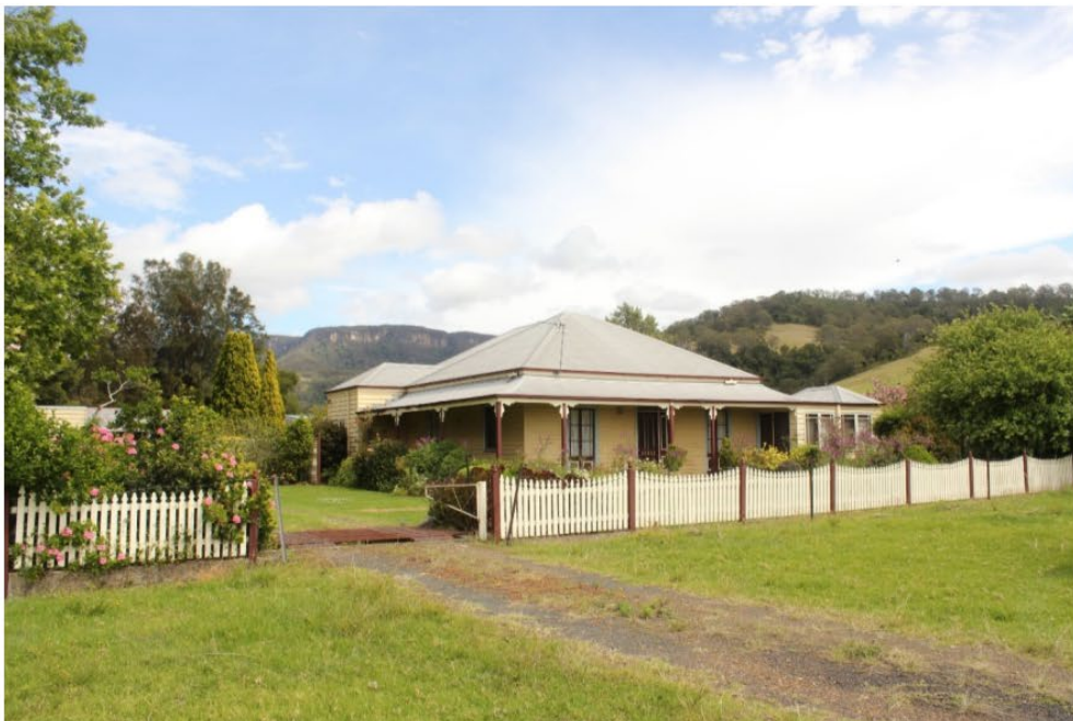
Figure 21: Miala showing the picket fence and garden setting of the house with escarpment backdrop behind. Note the cattle grate to the entry.
