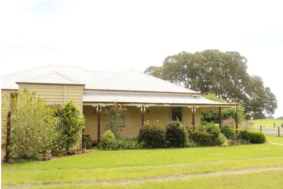
Figure 11: Southern façade of Miala cottage showing original veranda detail and original intact hipped roof form (right of image) and additions (left of image). Note the large established Fig.
