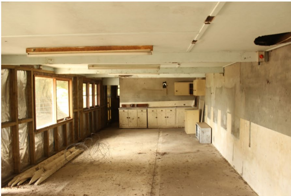
Figure 16: Interior of part of the dairy building, showing modifications including the filled in central milking pit.
