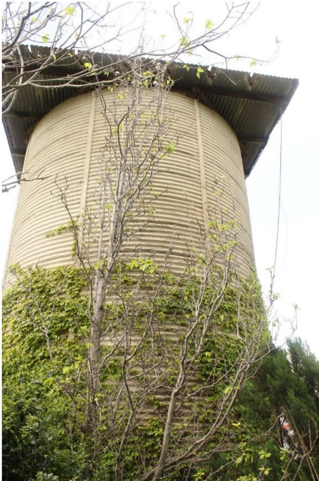
Figure 17: Detail of corrugated concrete silo located to the north west of the house. The flat roof structure tied to the ground with wires.
