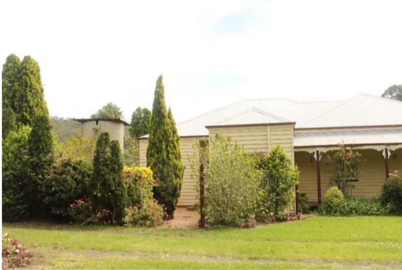
Figure 10: Southern façade showing recent additions to left of image, with the original veranda configuration and hopped roof form (right of image). Note the position of the silo to far left.
